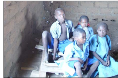
Students study in a classroom in need of repair.
